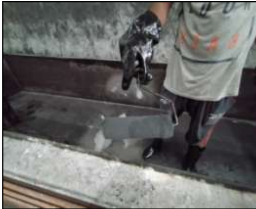
Fig 6.5: Use of the Roller Brush for Applying Oil
