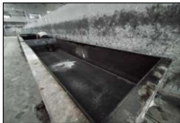
Fig 6.3: Mold without Oil Coating
